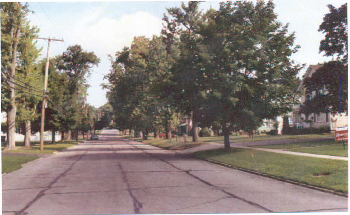
August 8, 2003 South Vernon Street Pre-Construction Looking North
